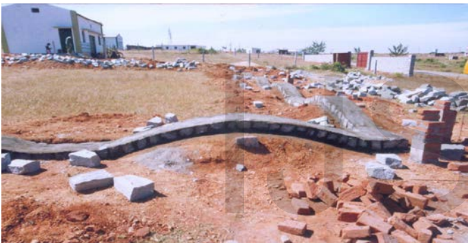
Plate 4. Construction of Arches in foundations
