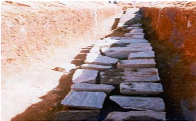
Plate 3. Placing of boulders over cement concrete bed.
