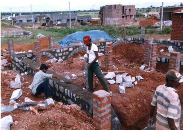
Plate 4. Construction of Arches in foundations
