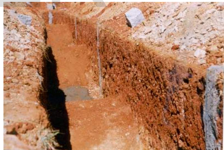
Plate 2. Excavation for Arch foundations
